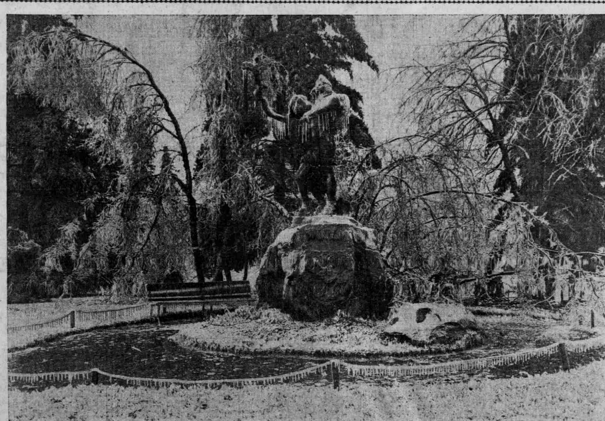
SCENE IN THE CITY PARK SHOWING THE WRECKAGE IN THE VICINITY OF THE "COMING OF THE WHITE MAN" STATUE.
