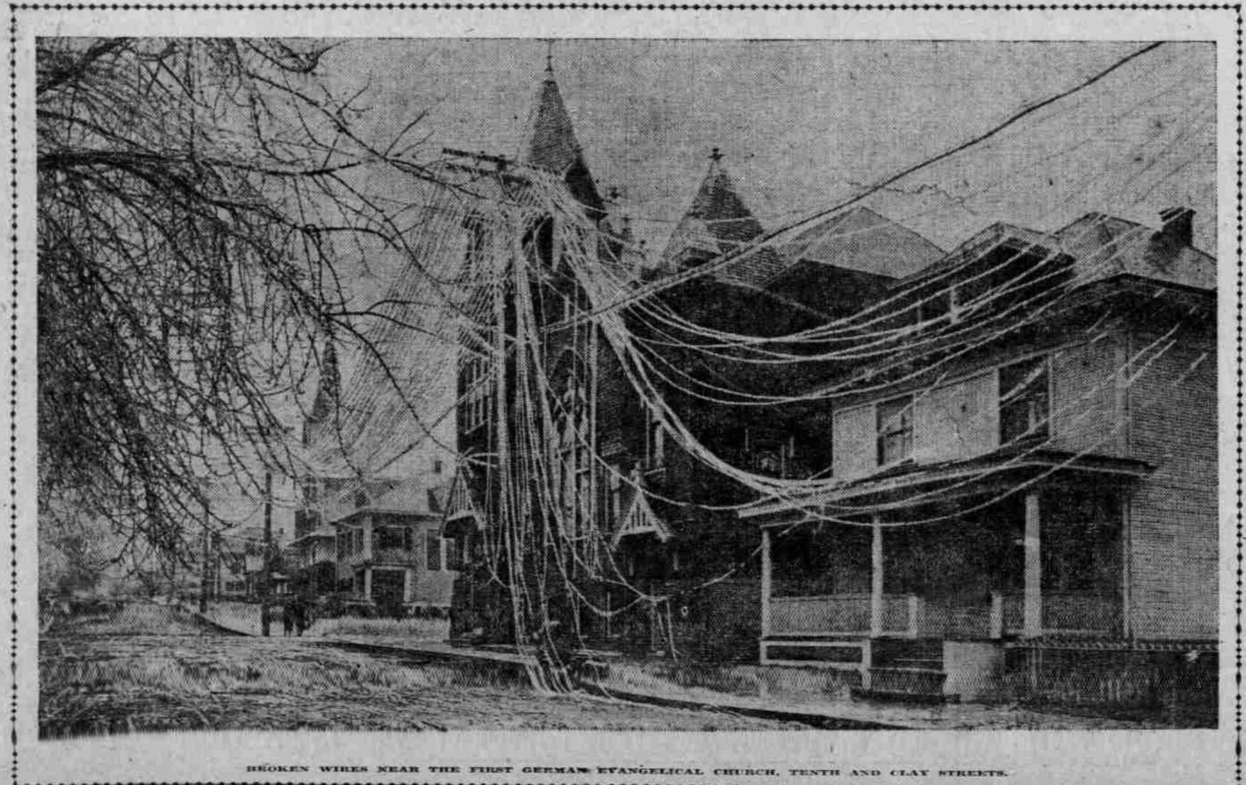
BROKEN WIRES NEAR THE FIRST GERMAN EVANGELICAL CHURCH, TENTH AND CLAY STREETS.
