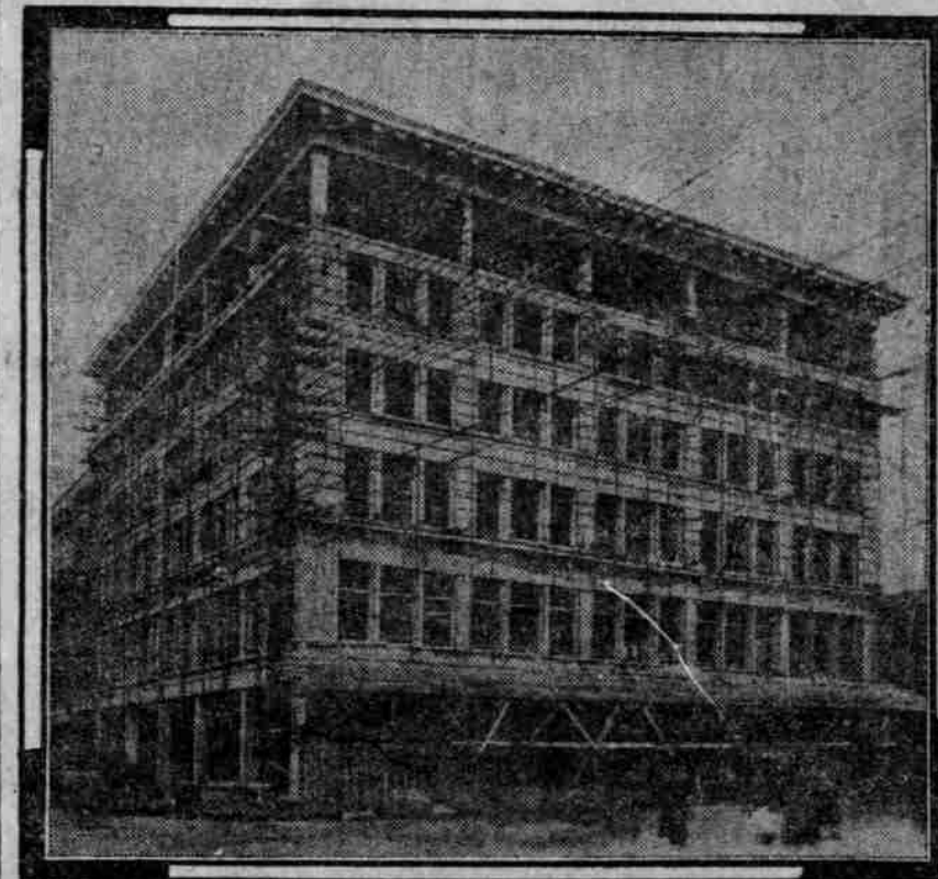
FALLING BUILDING 5TH AND ALDER
