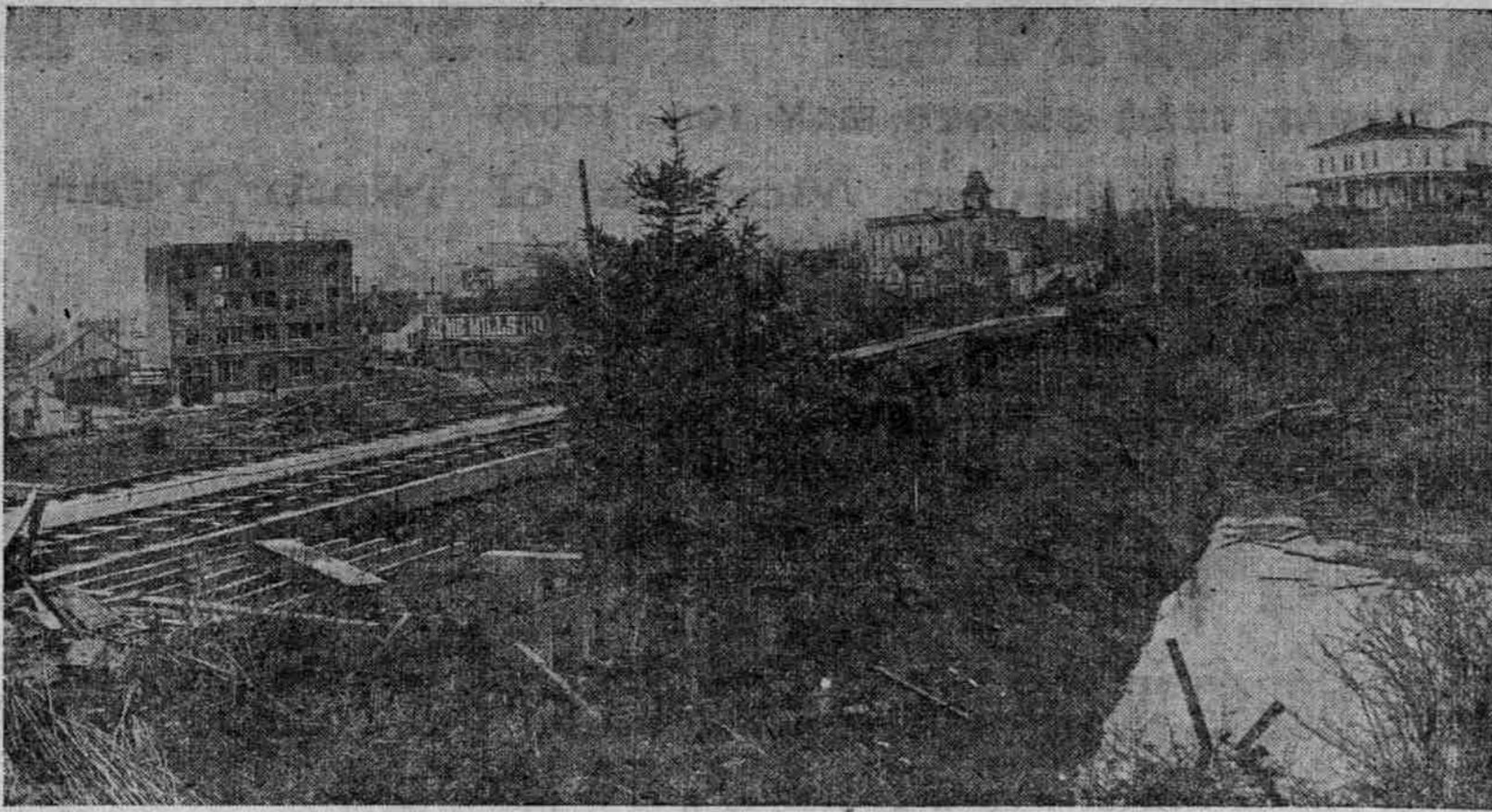
VIEW SHOWING FILL AT PRESENT STAGE OF OPERATIONS.
