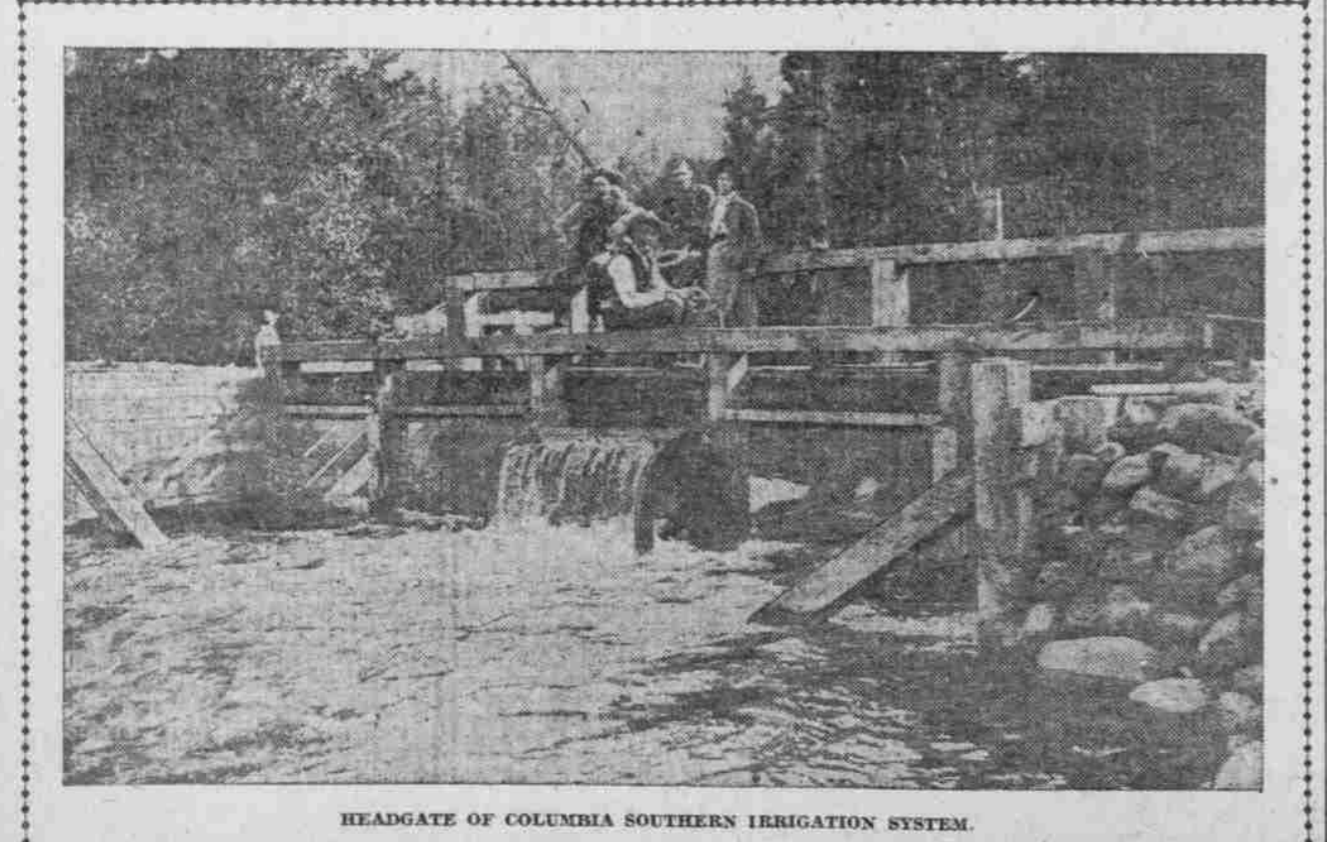
HEADGATE OF COLUMBIA SOUTHERN IRRIGATION SYSTEM.
