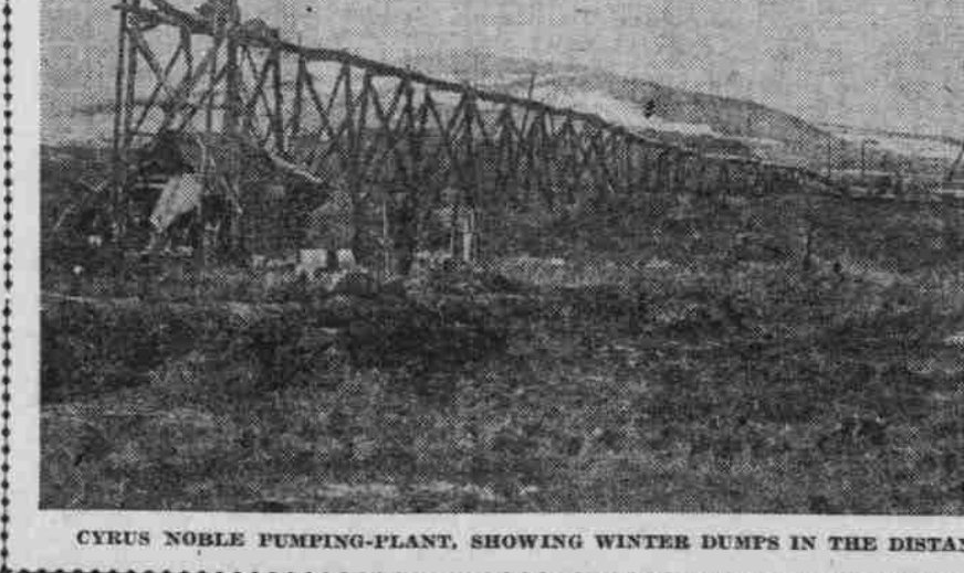
CYRUS NOBLE PUMPING-PLANT, SHOWING WINTER DUMPS IN THE DISTANCE—NOME, ALASKA, MAY 23, 1906.
