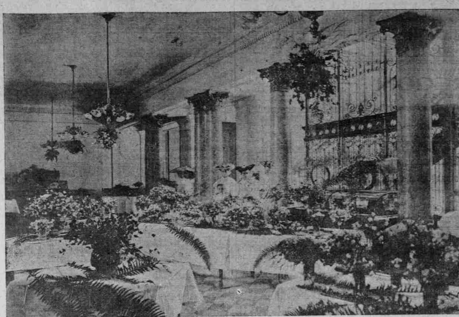
EXHIBIT ON THIRD FLOOR OF CITY HALL.
