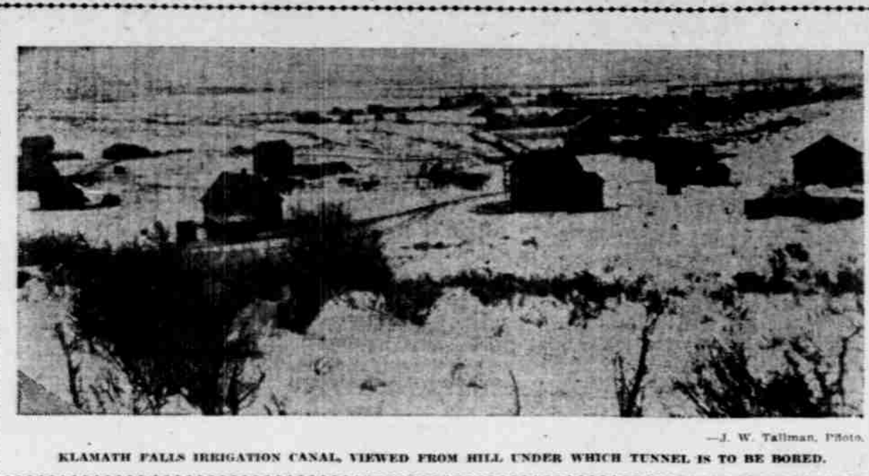
KLAMATH FALLS IRRIGATION CANAL, VIEWED FROM HILL UNDER WHICH TUNNEL IS TO BE BORED.
