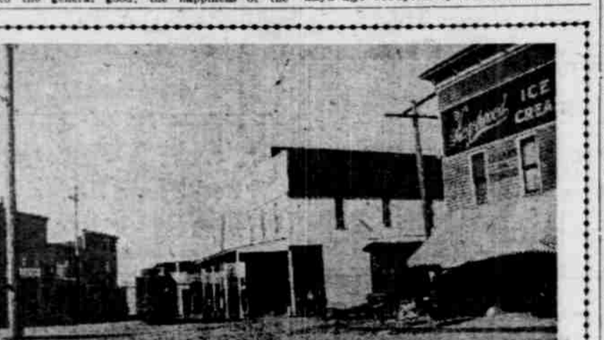
ON THE RIGHT IS SHOWN THE HAZELWOOD CONFECTIONERY STORE, WHICH WAS DESTROYED. FOUR BUILDINGS TO THE RIGHT WERE ALSO BURNED TO THE GROUND. BUILDINGS IN FOREGROUND WERE ENDANGERED.
