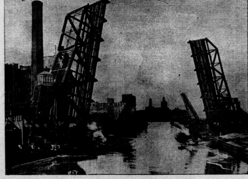
DOUBLE-TRACK SCHERZER ROLLING LIFT BRIDGE OVER THE CRICAGO RIVER AT THE ENTRANCE TO THE GRAND CENTRAL STATION, CHICAGO, The length of the span of this bridge in the clear is 275 feet, and the river is so narrow that a swing bridge pier for a structure of this size would practiblockade the channel. This condition does not have to be contended with in the Willamette, where the channel can be widened to six or seven times the width of the river flowing through Chicago.
