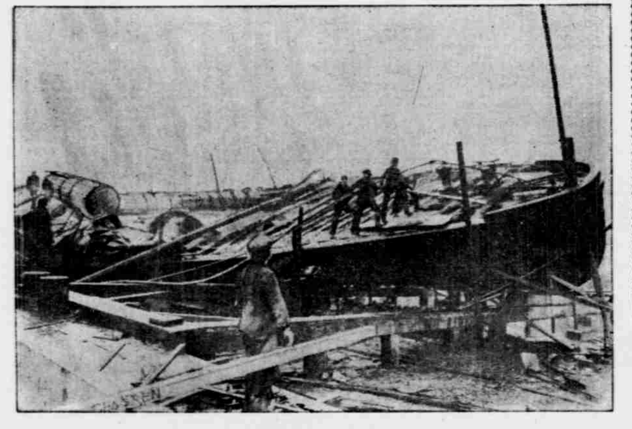
FORWARD PART OF STEAMER REGULATOR, SHOWING HOLE IN THE SIDE (TO RIGHT OF THE BOY) THROUGH WHICH FIREMAN STAYTON WAS BLOWN BY THE FORCE OF THE EXPLOSION.
