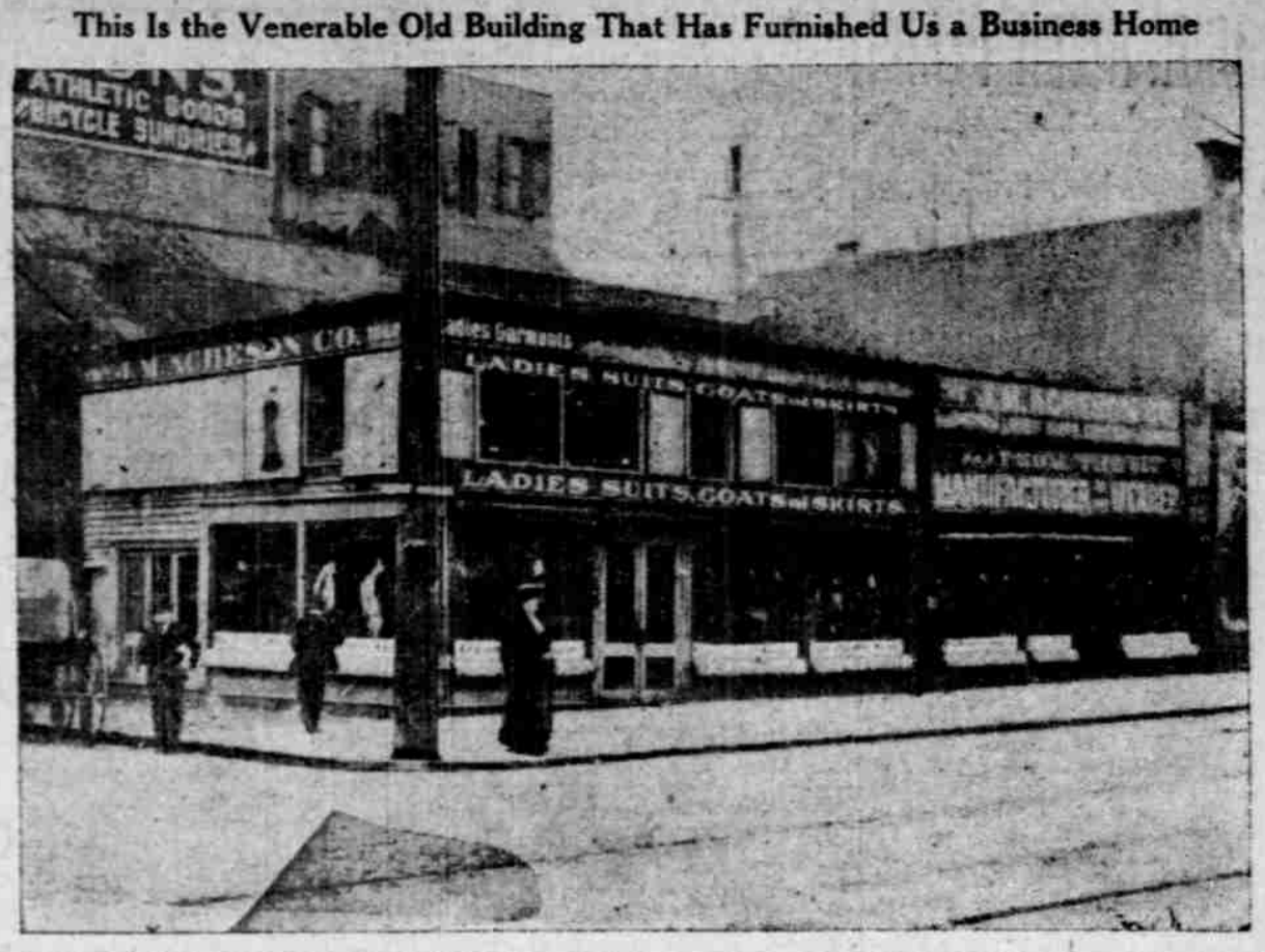
This Is the Venerable Old Building That Has Furnished Us a Business Home
