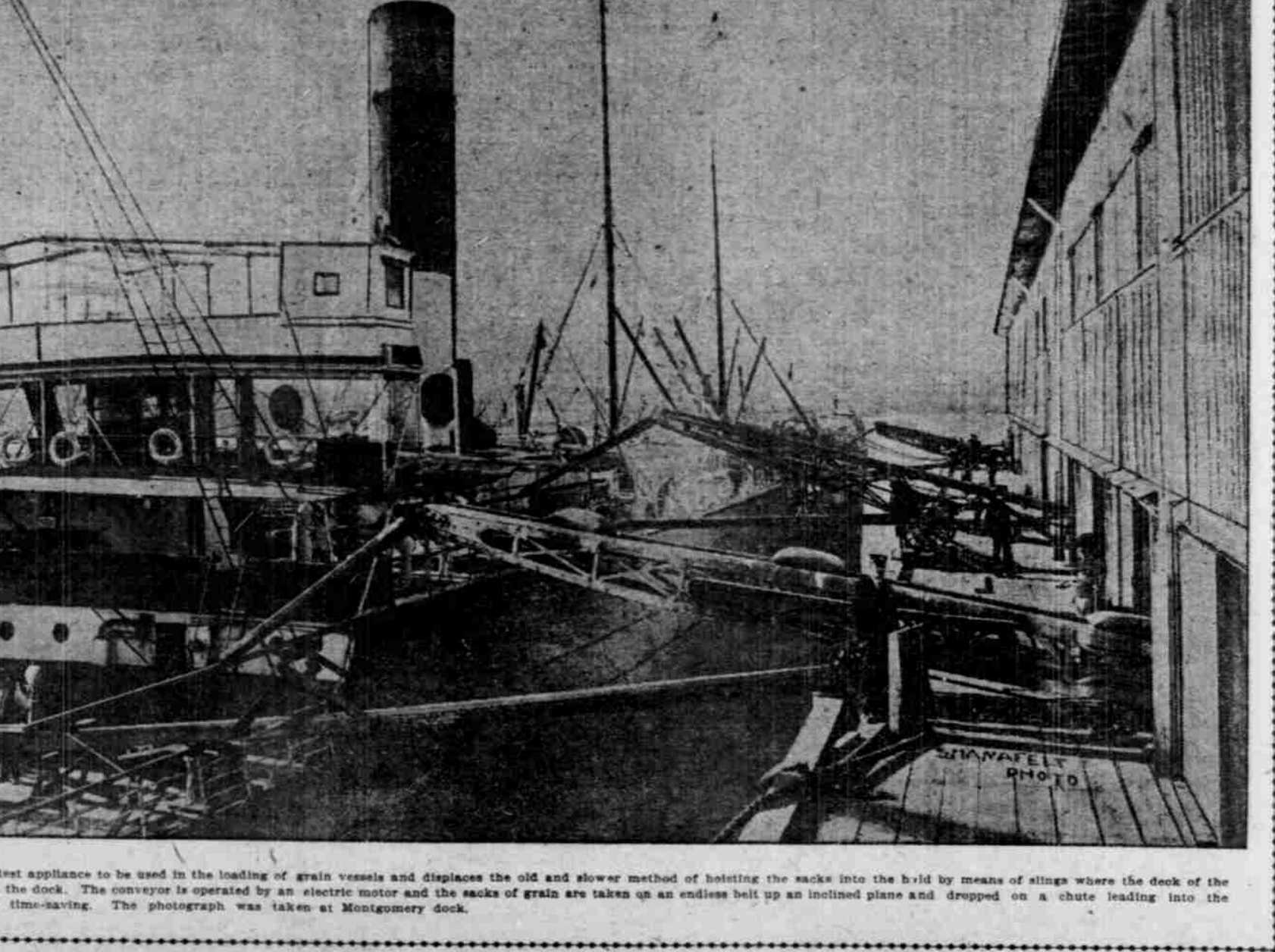
The electric conveyor is the latest appliance to be used in the loading of grain vessels and displaces the old and slower method of hoisting the sacks into the hold by means of slings where the deck of the vessel is on a level with or higher than the dock. The conveyor is operated by an electric motor and the sacks of grain are taken up an endless belt up an inclined plane and dropped on a chute leading into the hatch. Its one great feature is that of time-saving. The photograph was taken at Montgomery dock.
