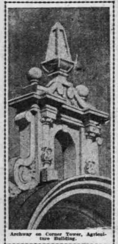
Archway on Corner Tower, Agriculture Building.
