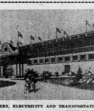
MACHINERY, ELECTRICITY AND TRANSPORTATION BUILDING.
