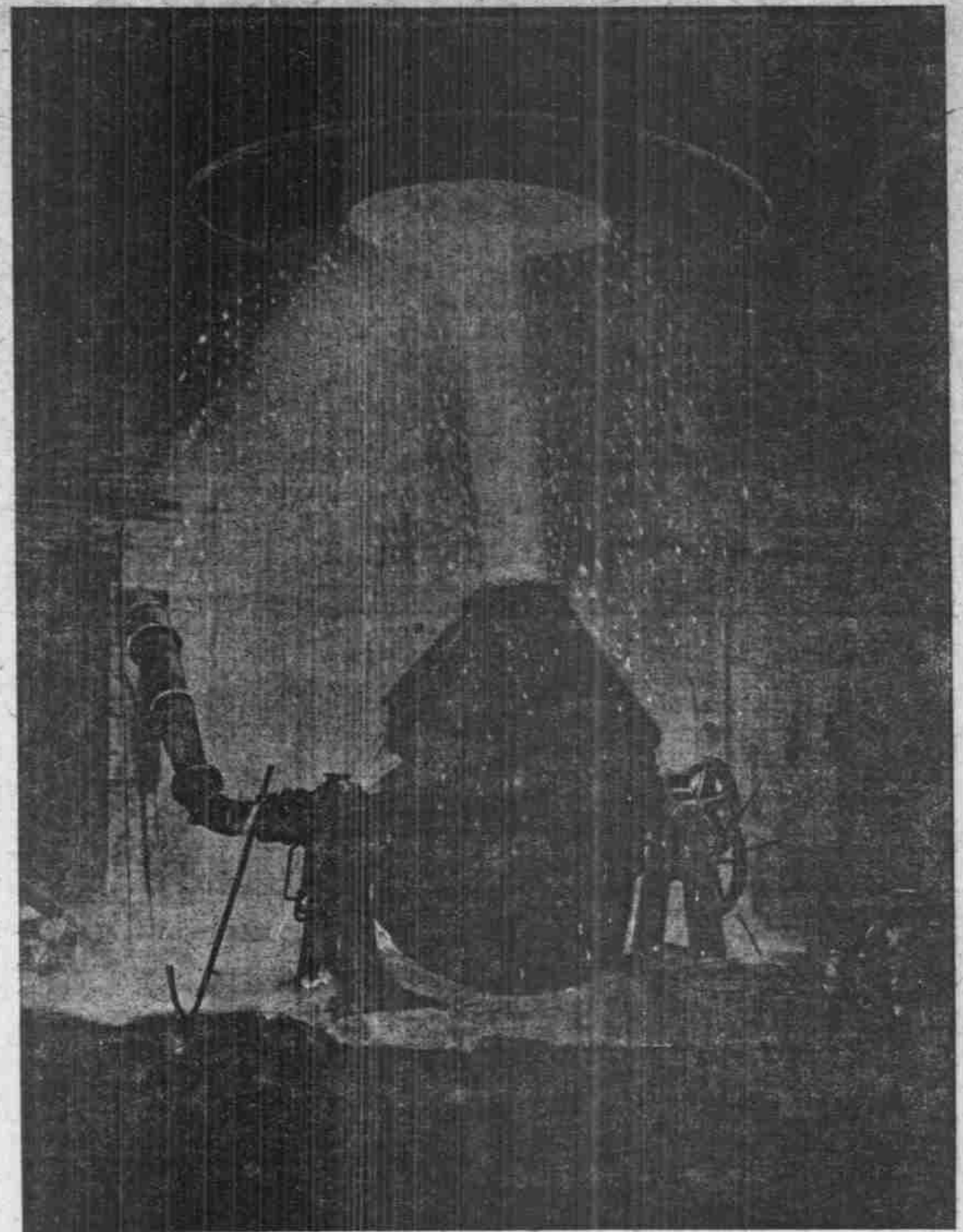
TWO-TON CONVERTER UNDER BLAST Steel Dept., Columbia Engineering Works.
