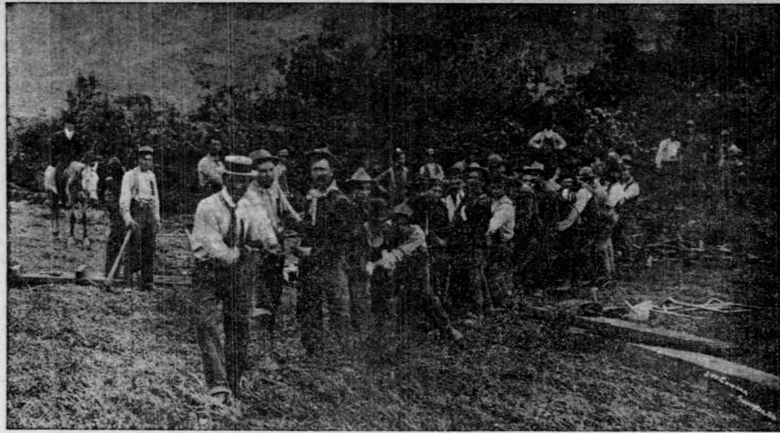
THE BAKER CITY-SUMMIT RELIEF CREW OPENING A DRIFT FOUR MILES BELOW HEPPNER. THE BRUSH BACK OF THE MEN IS ONE MASS OF WRECKAGE FROM DEMOLISHED BUILDINGS.
