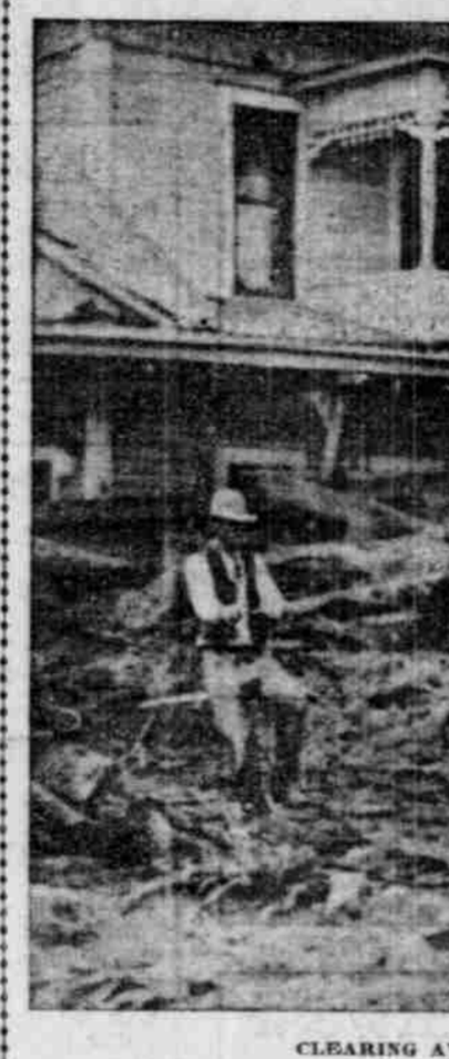
CLEARING AWAY THE DEBRIS OF A WRECKED BUILDING
