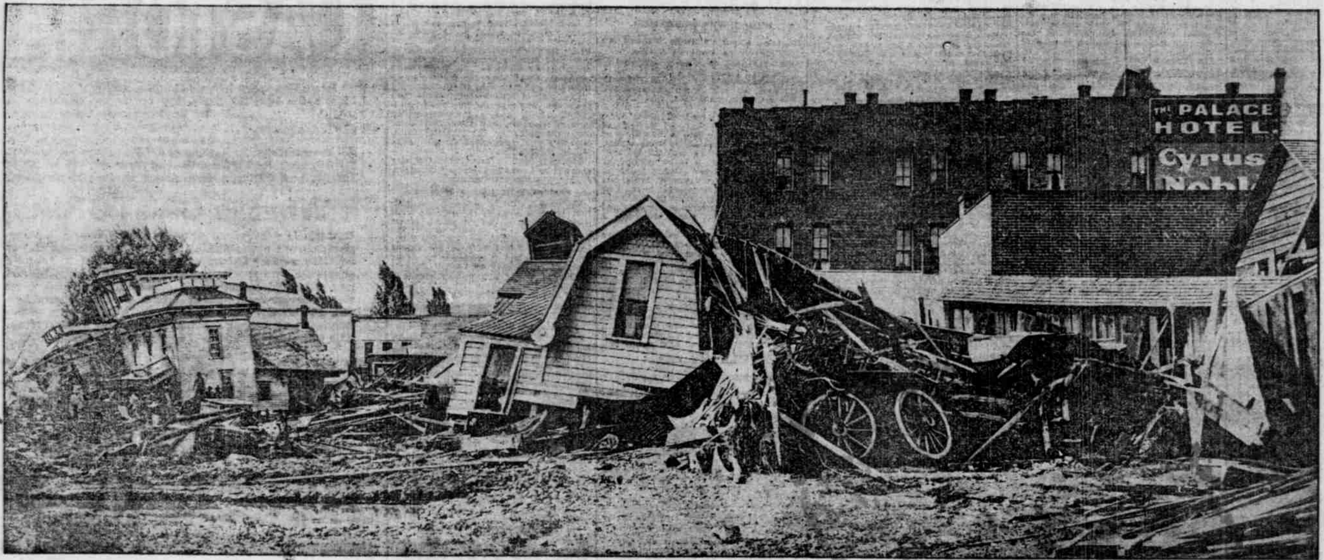
WRECKAGE OF THE RESIDENCES OF SHERIFF SHURT AND THOMAS AYERS IN PATH OF THE FLOOD.
