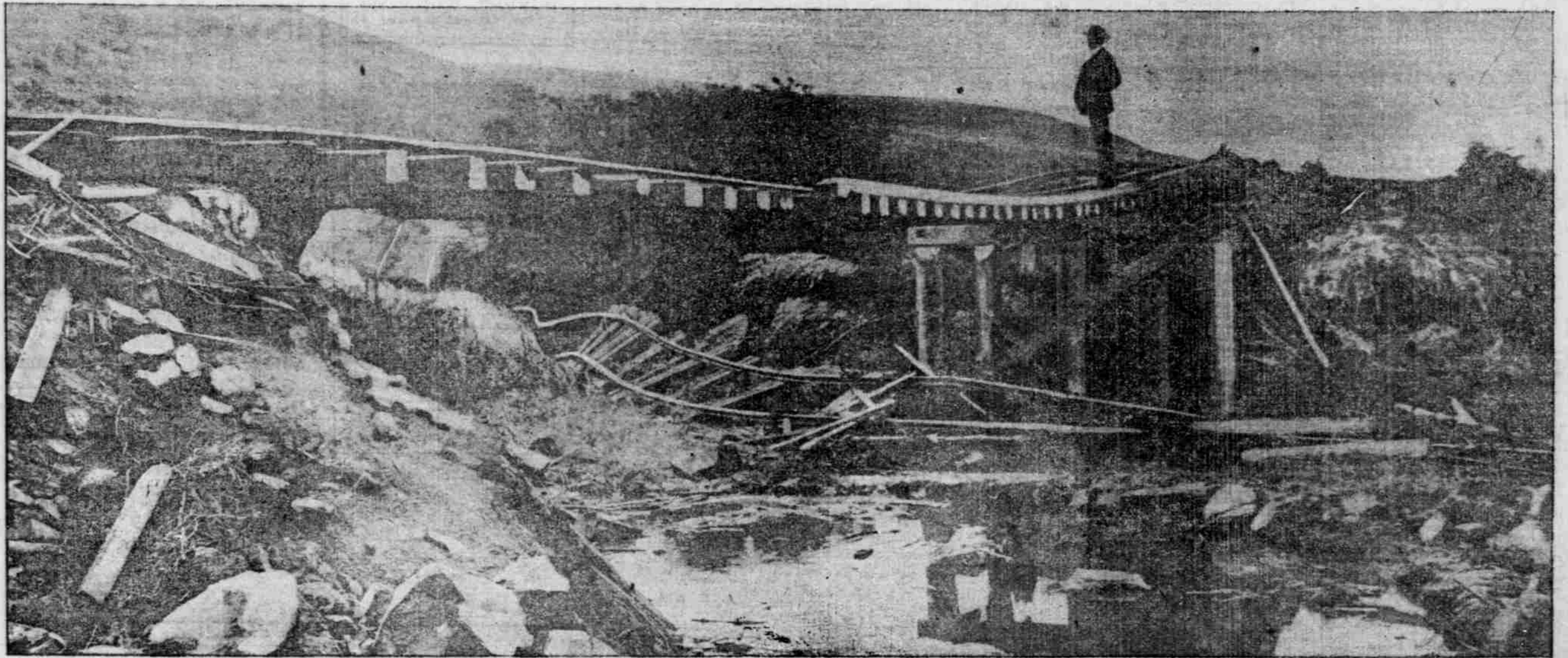
FIRST WRECKED BRIDGE OVER WILLOW CREEK ON O. R. & N. LINE, A FEW MILES BELOW LEXINGTON.
