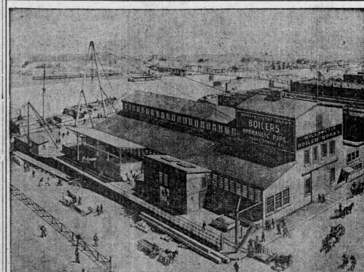
WILLAMETTE BOILER WORKS FRONT AND EVERETT STREETS, PORTLAND, OR.
