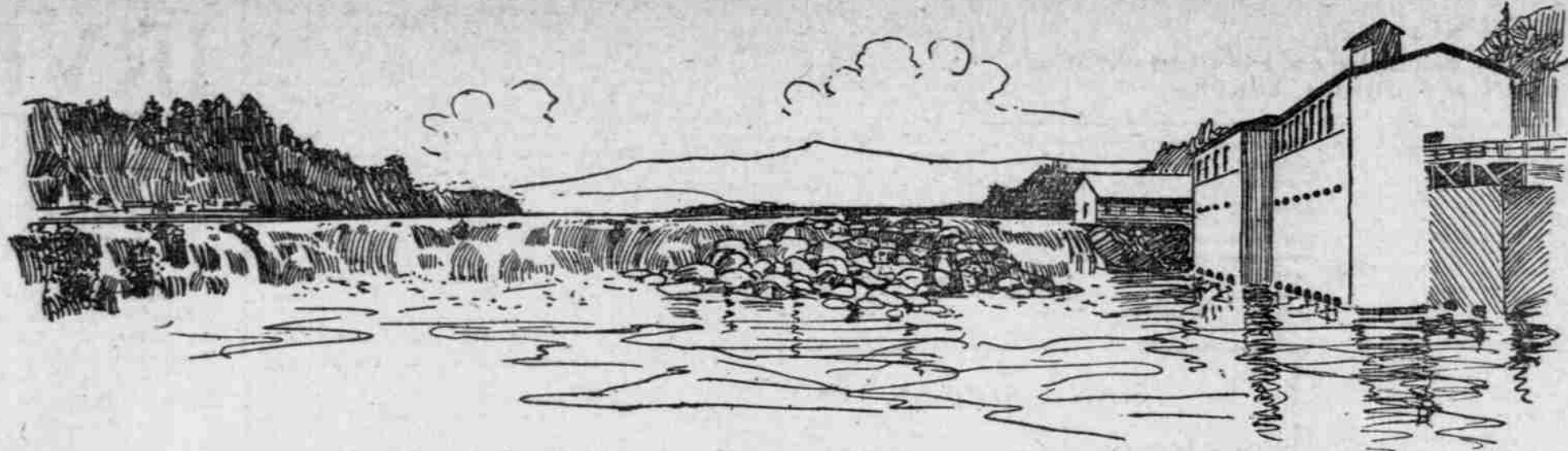
Portland General Electric Co.'s Generating Station B at Willamette Falls, Present Capacity 10,000 Horse-Power, Under Construction 4,000 Additional Horse-Power
