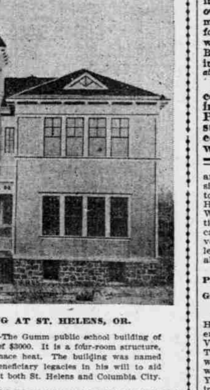
NEW PUBLIC SCHOOL BUILDING AT ST. HELENS, OR.
