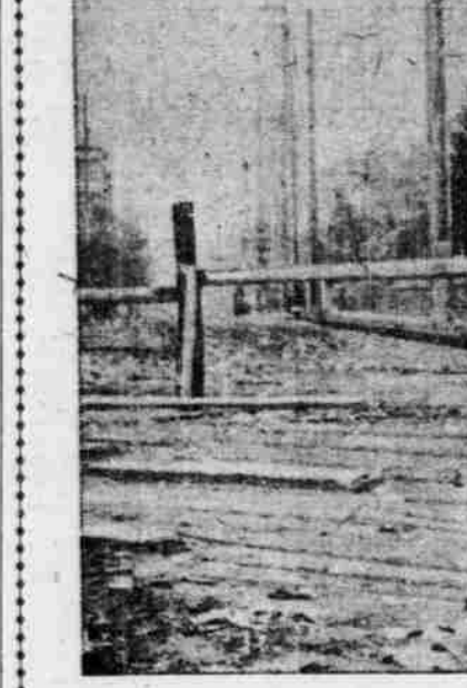
VIEW OF ALDER-STREET ROADWAY.
