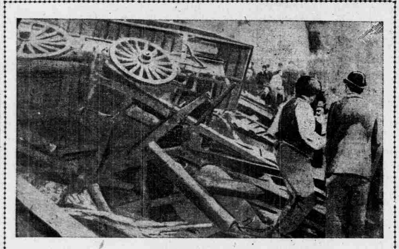
IN THE DEBRIS OF THE COLLAPSED MARQUAM GULCH BRIDGE.
