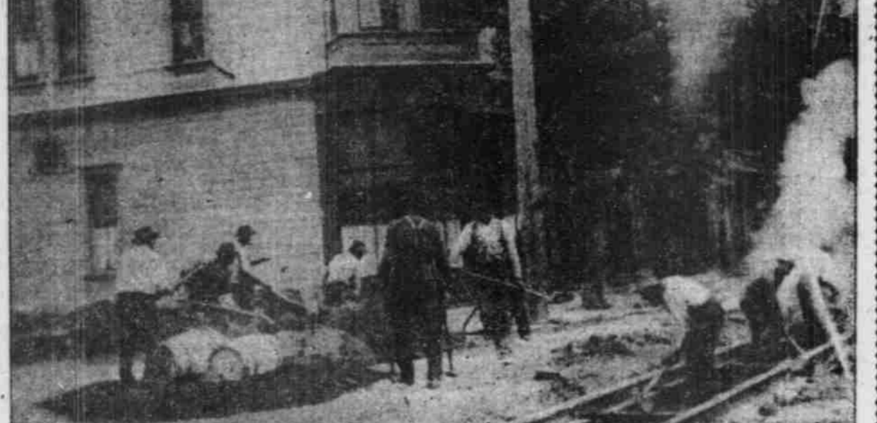
WELDING THE HEAVY STEEL RAILS BY ELECTRIC PROCESS.
