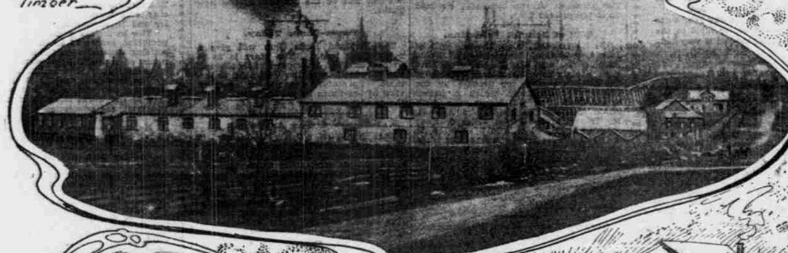
MAIN MACHINE BUILDINGS
