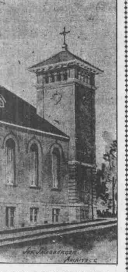
The above picture shows the new St. Michael's Italian Church, on the southwest corner of Fourth and Mill streets, will appear when the structure is completed.
