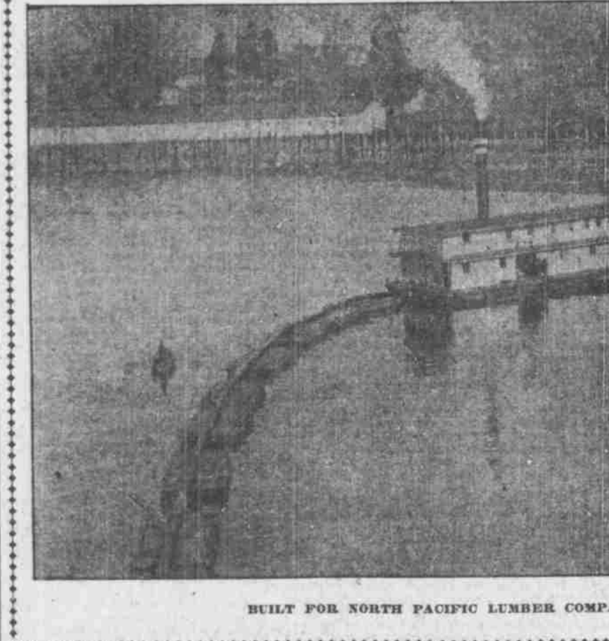
BUILT FOR NORTH PACIFIC LUMBER COMPANY.
