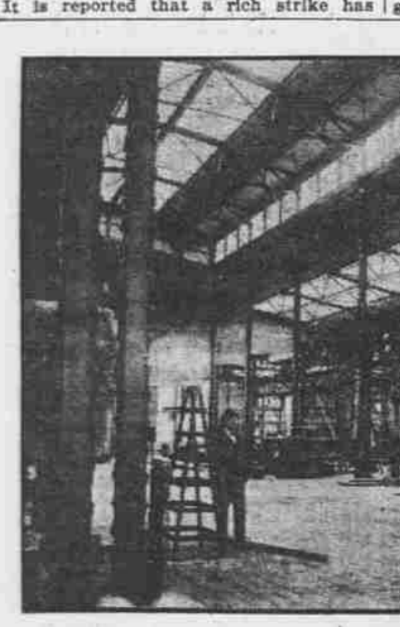
SOUTHERN PACIFIC SHOPS—INTERIOR.
