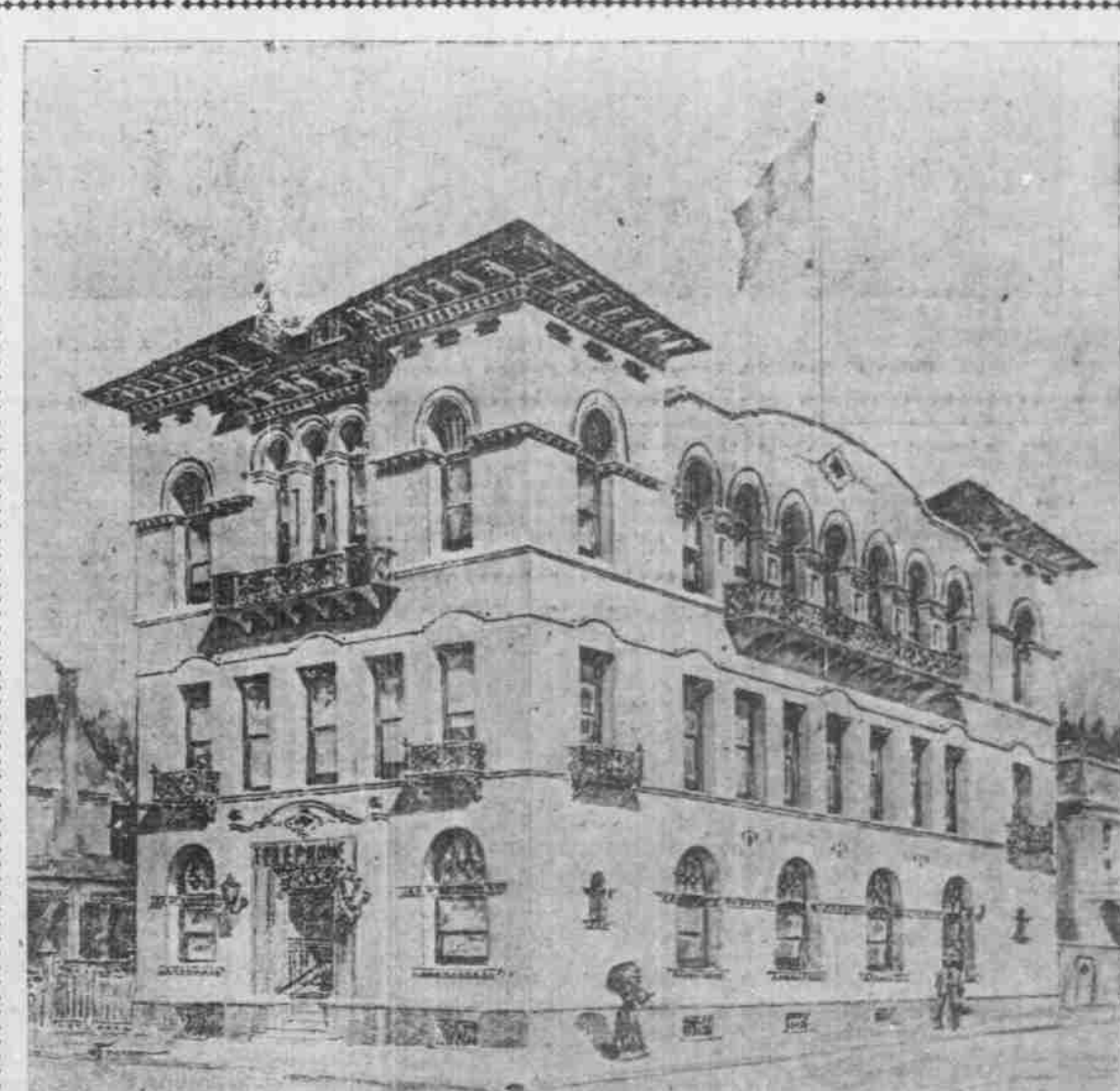
THE NEW HEADQUARTERS BUILDING OF THE PACIFIC STATES TELEPHONE & TELEGRAPH COMPANY, PORTLAND, OR.
