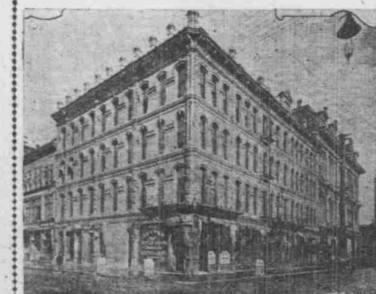
THE "LOUVRE" AND HOTEL BELVEDERE. Fritz Strobel & Co., Props. N. E. Cor. Alder and Fourth Sts.
