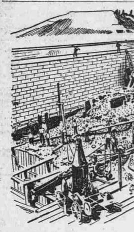
THE NEW LOCKS IN THE YAMHILL RIVER—EXCAVATING FOR FOUNDATION OF DAM.
