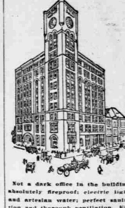
Not a dark office in the building; absolutely fireproof; electric lights and artesian water; perfect sanitation and thorough ventilation. Elevators run day and night.
