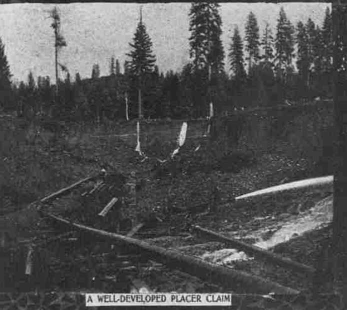
TWO 8-INCH GIANTS PLAYING ON A 40-FOOT BANK OF GRAVEL
