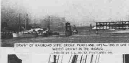
—PHOTO BY J. H. BATH, PORTLAND, OR. DRAW OF RAILROAD STEEL BRIDGE PORTLAND, OREG.—THIS IS ONE OF THE WIDEST DRAWN IN THE WORLD.
