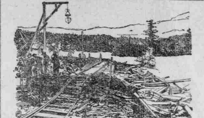
WORKING ON UPPER BULKHEAD, JUNE 4, 1881.
