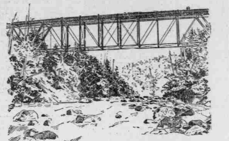
RESERVOIR NO. 1, ACROSS BULL RUN BELOW HEAD WORKS.—Photo. by Towne.
