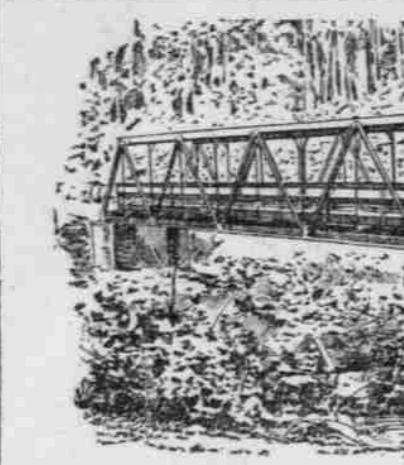
RESERVOIR NO. 1, ACROSS BULL RUN BELOW HEAD WORKS.—Photo. by Towne.
