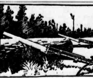
SAWING WITH COMPRESSED AIR.
