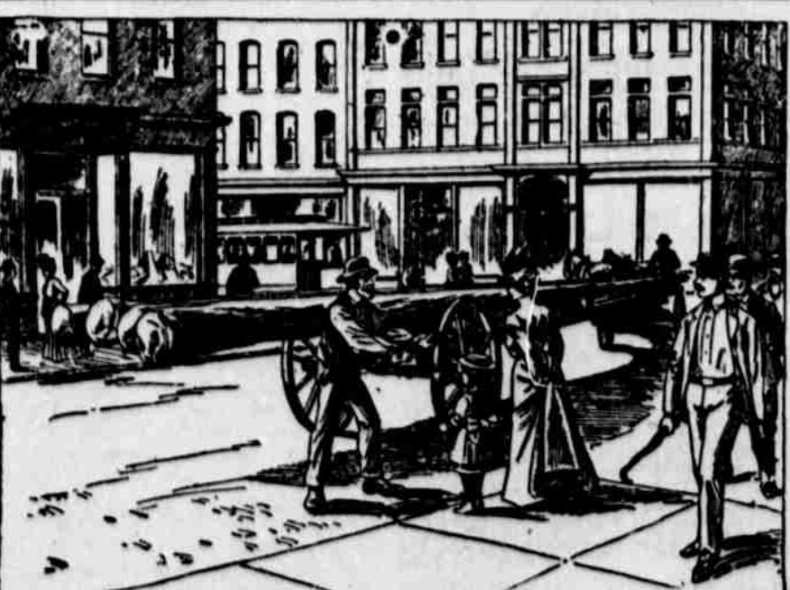
PILOTING LONG POLES THROUGH THE STREETS.
