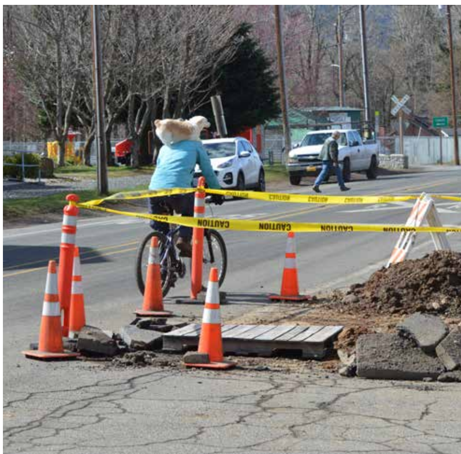
Pedestrians skirt cones surrounding road excavation on Baseline in Parkdale across from Lady Fern and Solera Brewery Wednesday. Parkdale Sanitary District issued a boil water order at 9 a.m. Wednesday, pending repairs, after a main line was exposed and a valve replaced. District officials said laboratory test results came back clean on Thursday at 3:30 p.m. and gave the okay to affected customers to use water as normal. (Under the order, water needed to be boiled when used for consumption or kitchen use and hygiene but not for bathing or clothes washing.) The order affected customers north of Baseline only.
