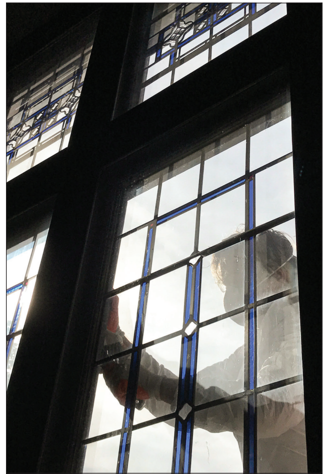
AUGUST: Michael Peterson repairs library window grout.
