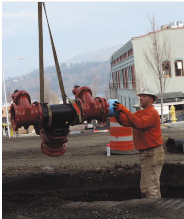
THIS PICTURE, a worker standing in a hole, putting something new into that hole — in this case a water line valve — best depicts the whole point of State Street Urban Renewal.
