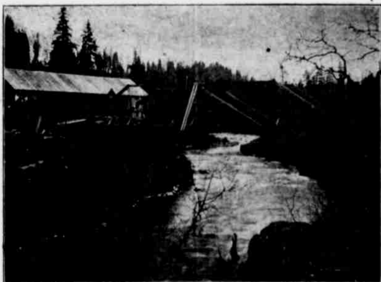
Hood River and Tucker's Bridge
