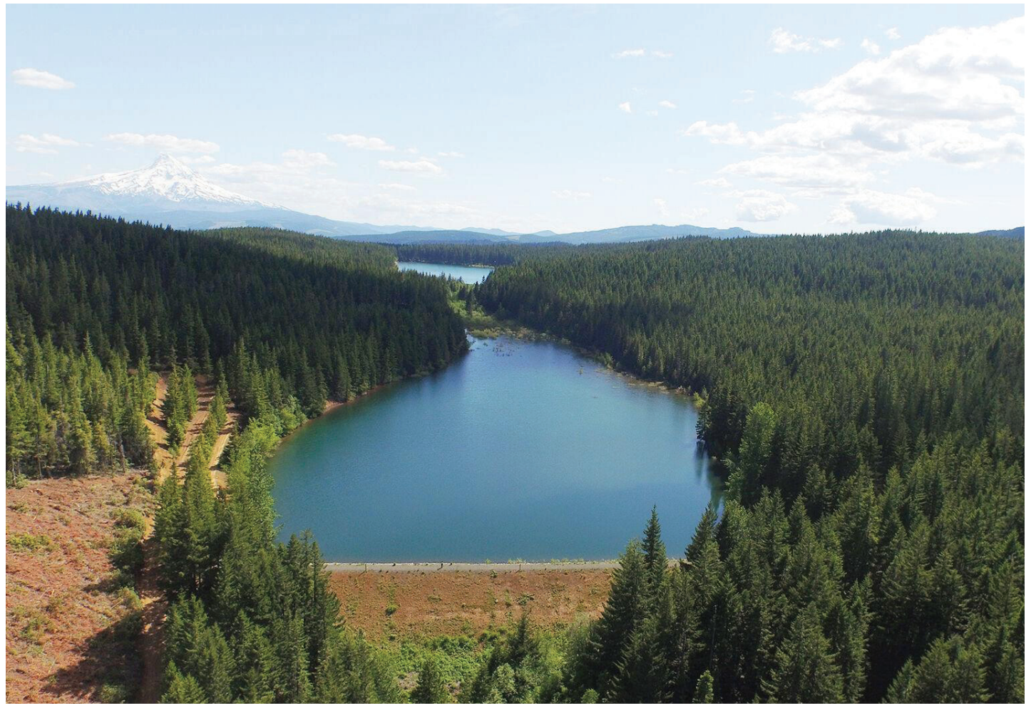
The Kingsley Dam near Hood River.
