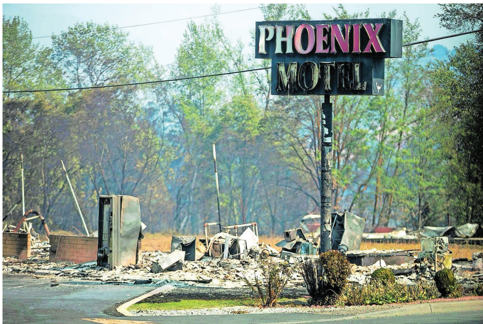
The remains of the Phoenix Motel in Phoenix after the Almeda fire in 2020.
