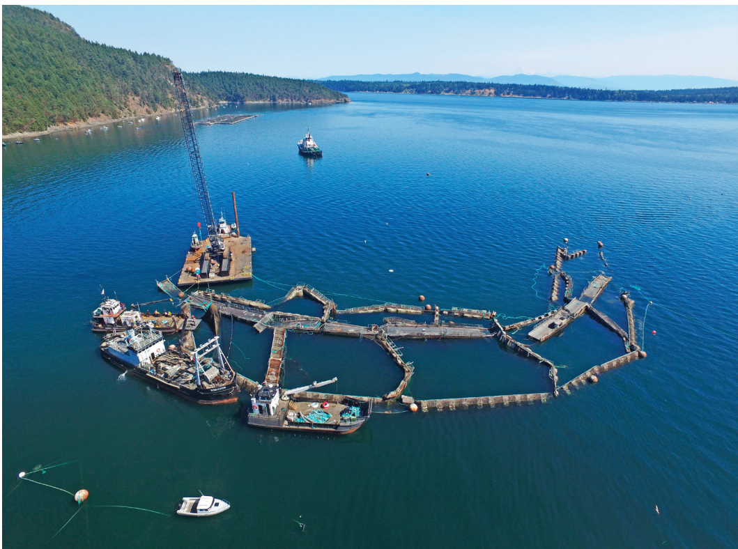
David Bergvall/Washington State Department of Natural Resources A crane and boats are anchored next to a collapsed net pen used by Cooke Aquaculture to farm Atlantic salmon near Cypress Island in Washington state in August 2017 after a failure of the nets allowed tens of thousands of the nonnative fish to escape.
