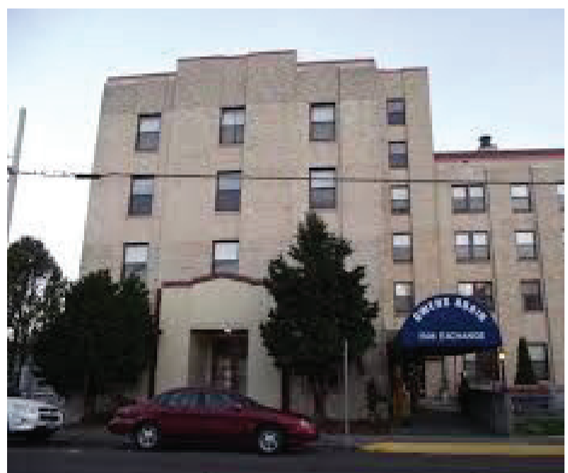
The sole elevator is out at the Owens-Adair near downtown.
