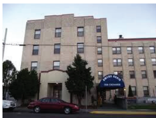
The elevator is down at the Owens-Adair Apartments.
