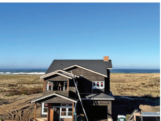
Ocean Front - Under Construction 1400 N Ocean Ave, Gearhart Craig & Dana Weston (503) 738-2838 $2,500,000
