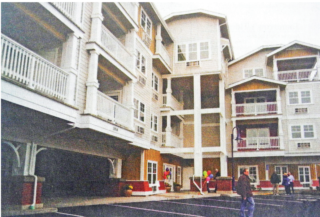
The city is examining code changes to allow more housing density.
